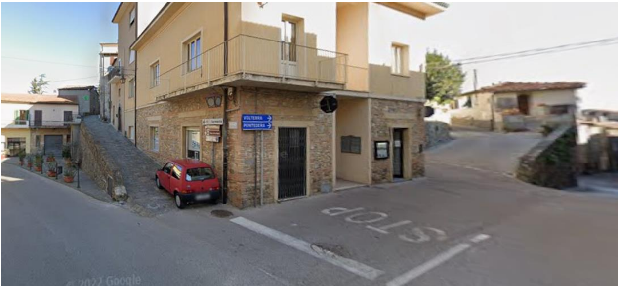
Figure 7 the two entrances to the church of San Donato, on the left from Via del Castello, on the right from the driveway
